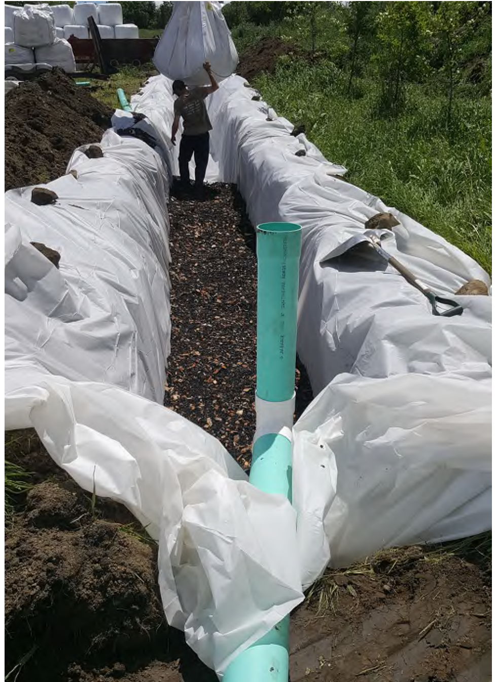
Churchill- Filter Installation
