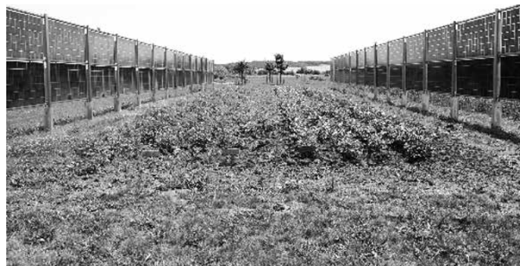
Vertical, bifacial solar arrays in a European agrovoltaic system.
