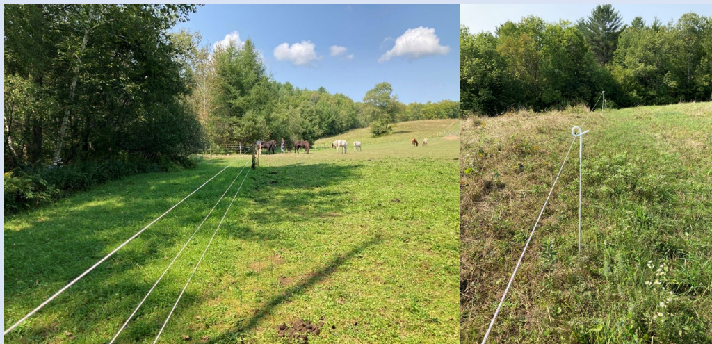
Figure 9. Newly installed perimeter fencing (left) which supports exclusion of livestock from surface water and pigtail fencing (right) with braided wire for temporary fencing between paddocks.
