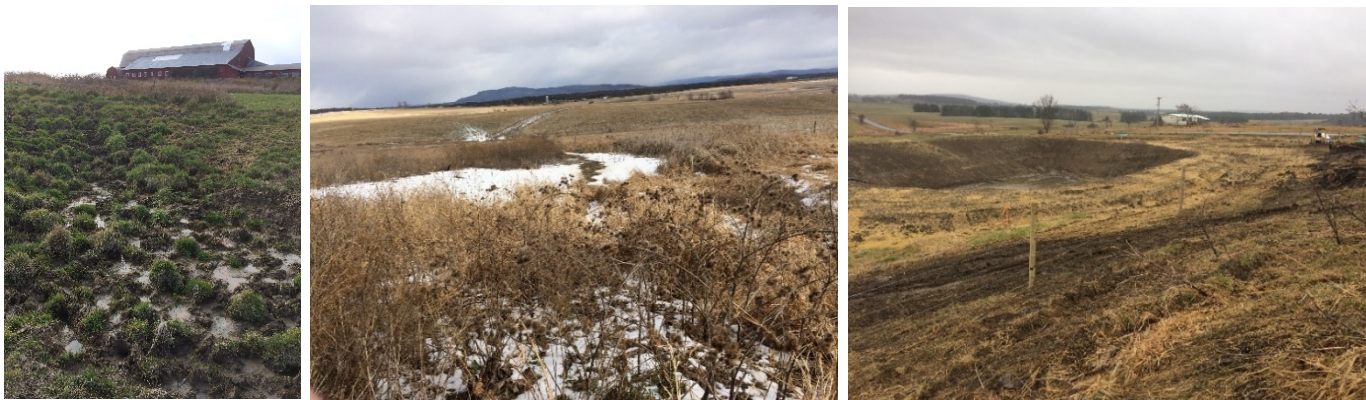
From left to right, before and after photos of waste storage facility installation to collect milkhouse wash water and manure
