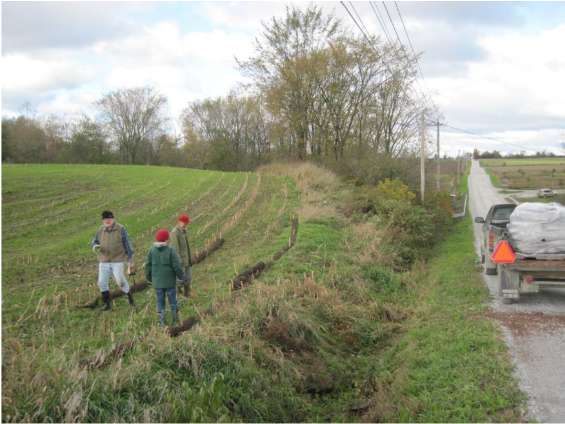
Even with well-vegetated buffer there is erosion in low spot where water funnels on its way to Rock River
