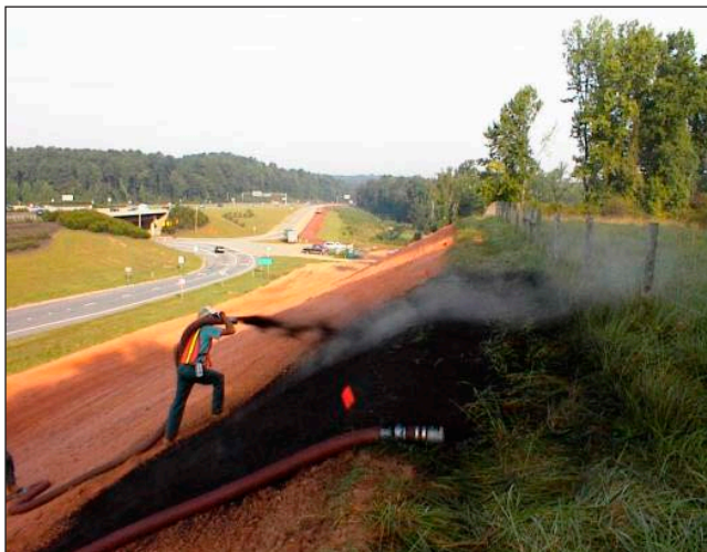
Figure 2 Slope application of compost blanket
