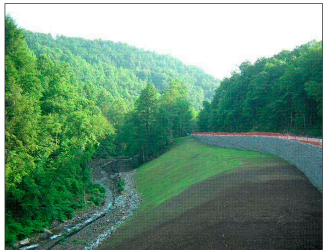
Figure 3 Establishing vegetation in a compost blanket
