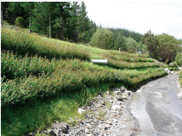
Figure 6 Vegetated compost filter socks
