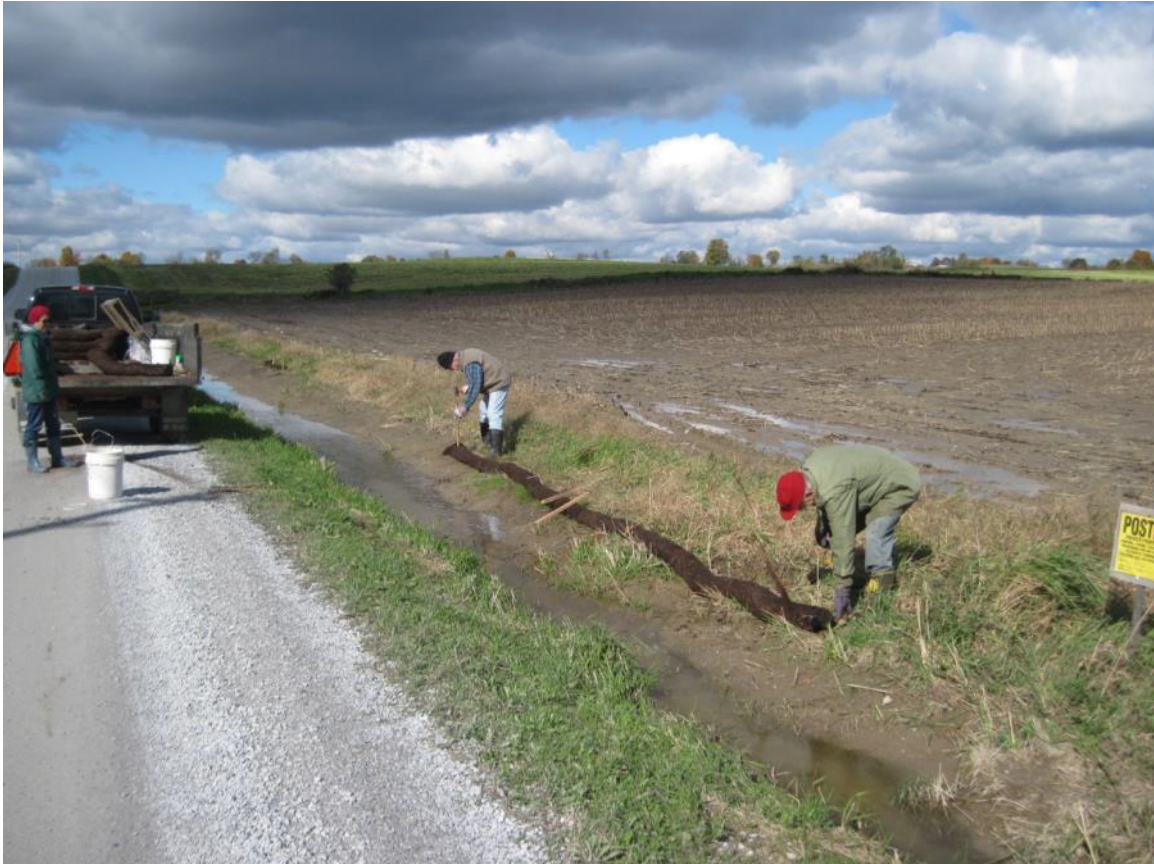
Compost Filter Sock can be used to reduce municipal ditch maintenance costs when the town's ditches abut cropland buffers with breaches. These breaches will become more of an issue with new regulations for towns under Act 64.
